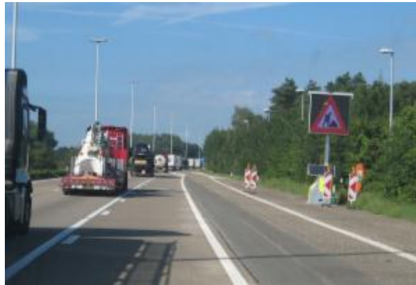
Mobile trailer with VMS (here 4400m before the work zone)
